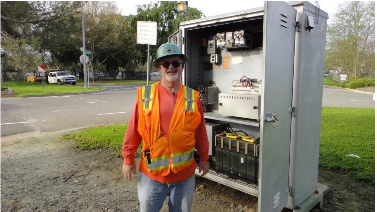
Signals AI deactivates the Front Street Grade Crossing Warning System so that the MOW Team's equipment can work within the circuit
