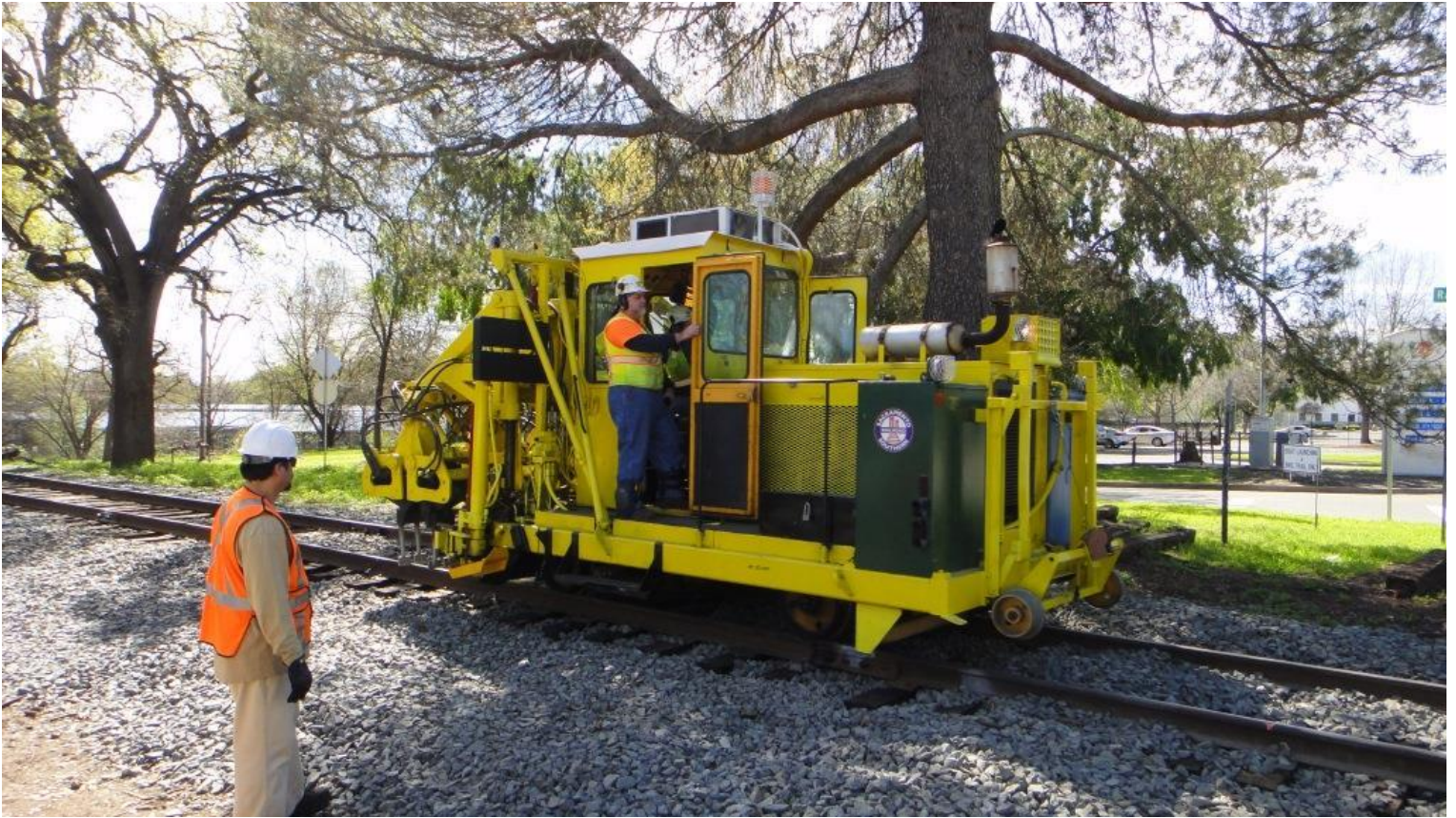
Heather and Mike F. run the tamper several times over the new track at maximum speed authorized under the rules
