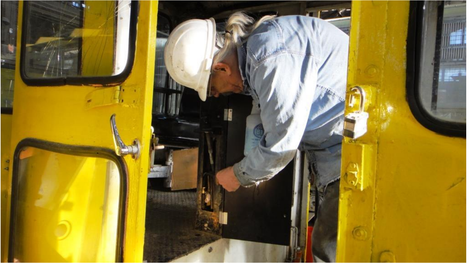
Fred locates a leak in the regulator's air system
