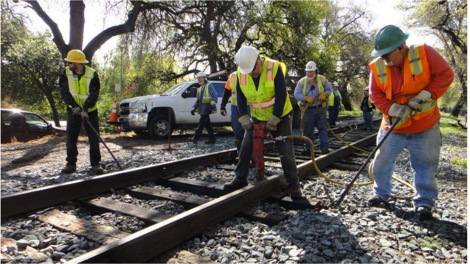
Musical spikers. Now Steve drives spikes while Chris M. and Al nip-up the tie and Frank guides the air-horse
