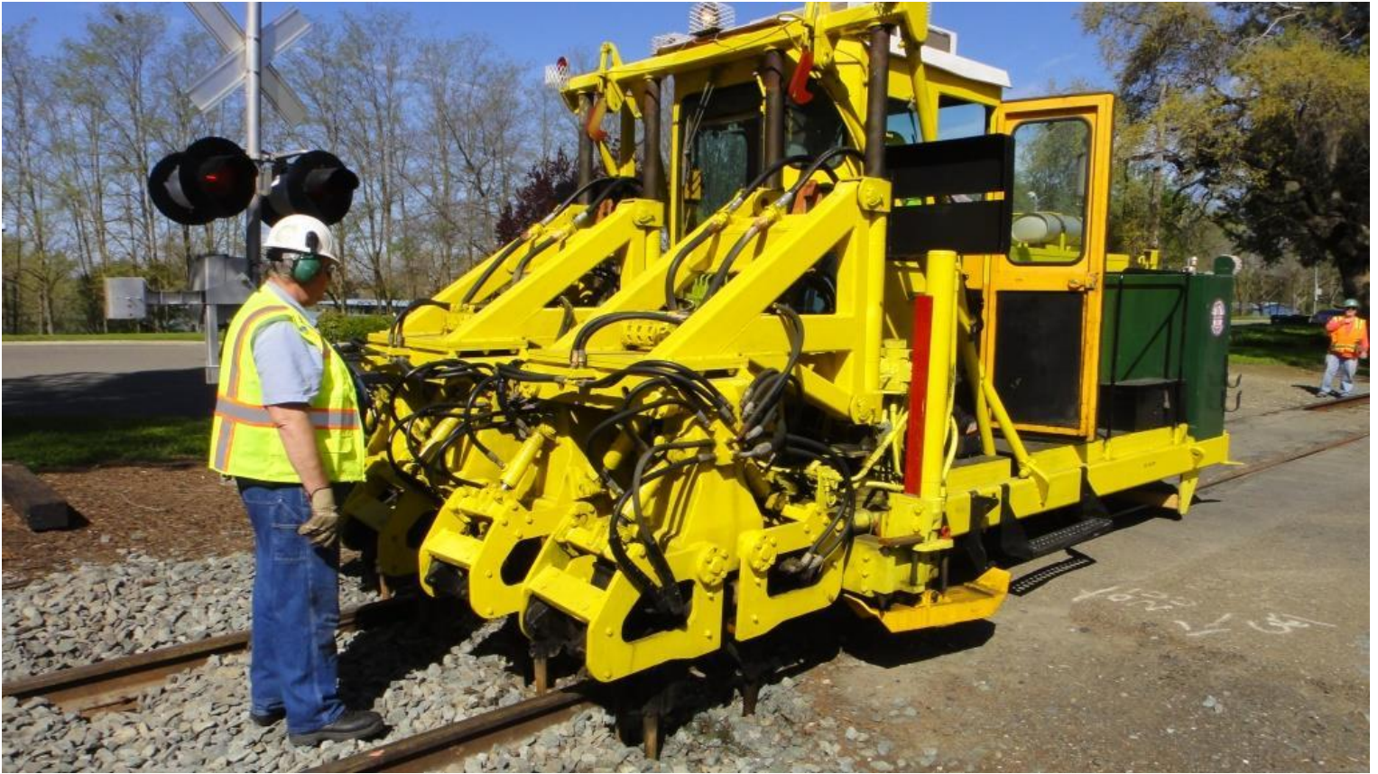
The very first tie south of the Front Street pavement is the first tie to be tamped-up
