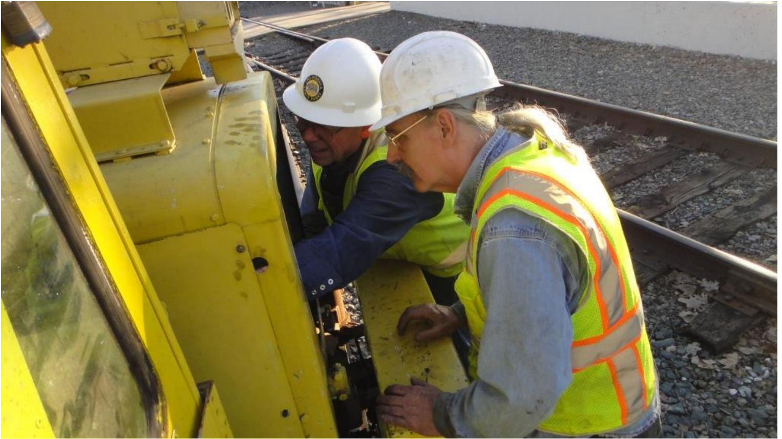
Cliff and Fred install the new governor on the scarifier's air-compressor
