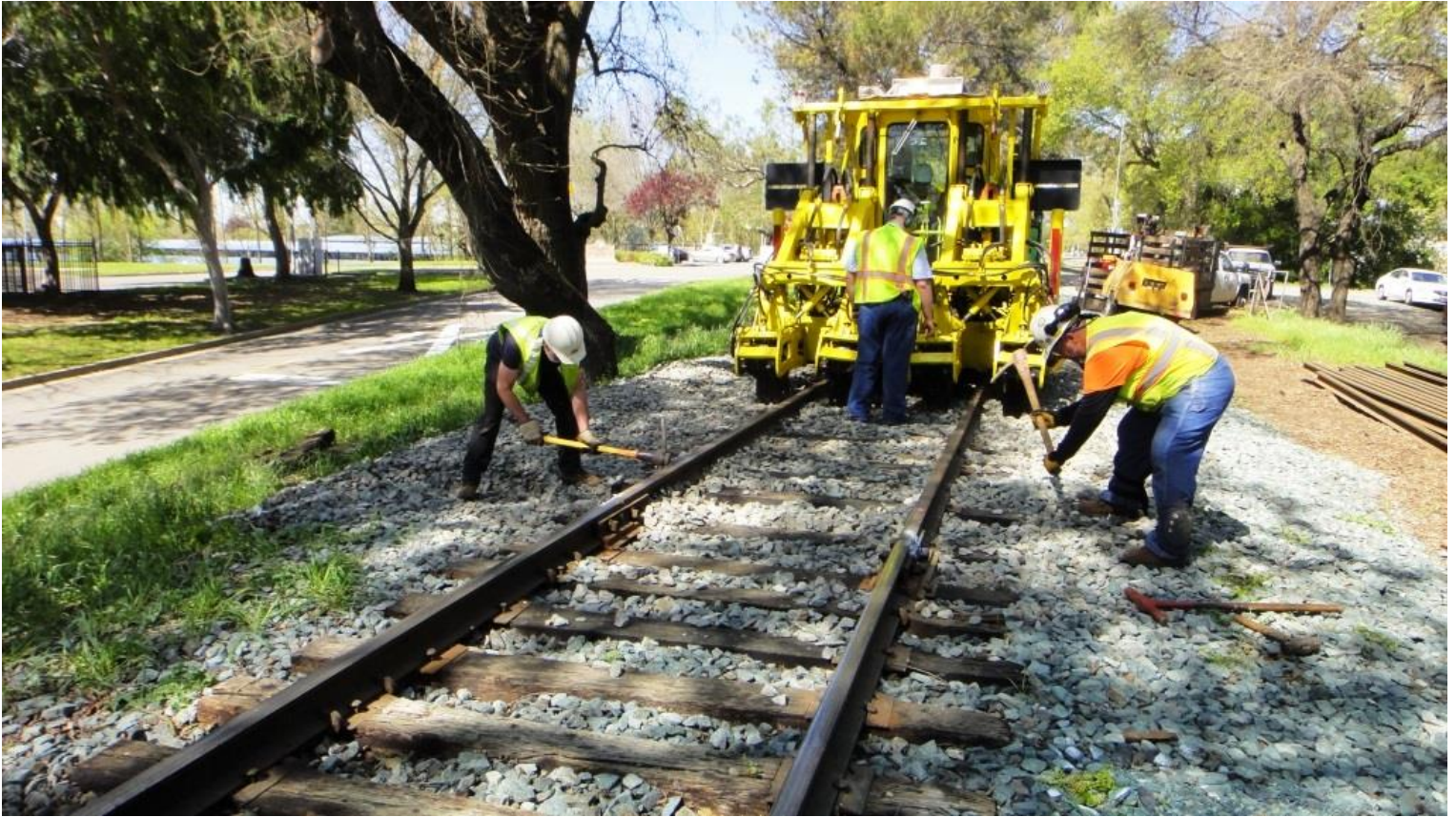
Mike M. and Mike F. loosen some ballast so that the tamper can be used to shove a tie a few inches south
