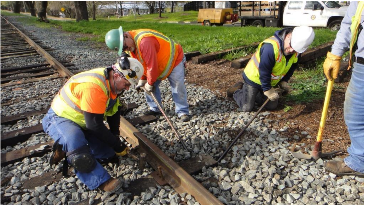
Al and Steve double-up the nipping power as Mike F. sets a spike
