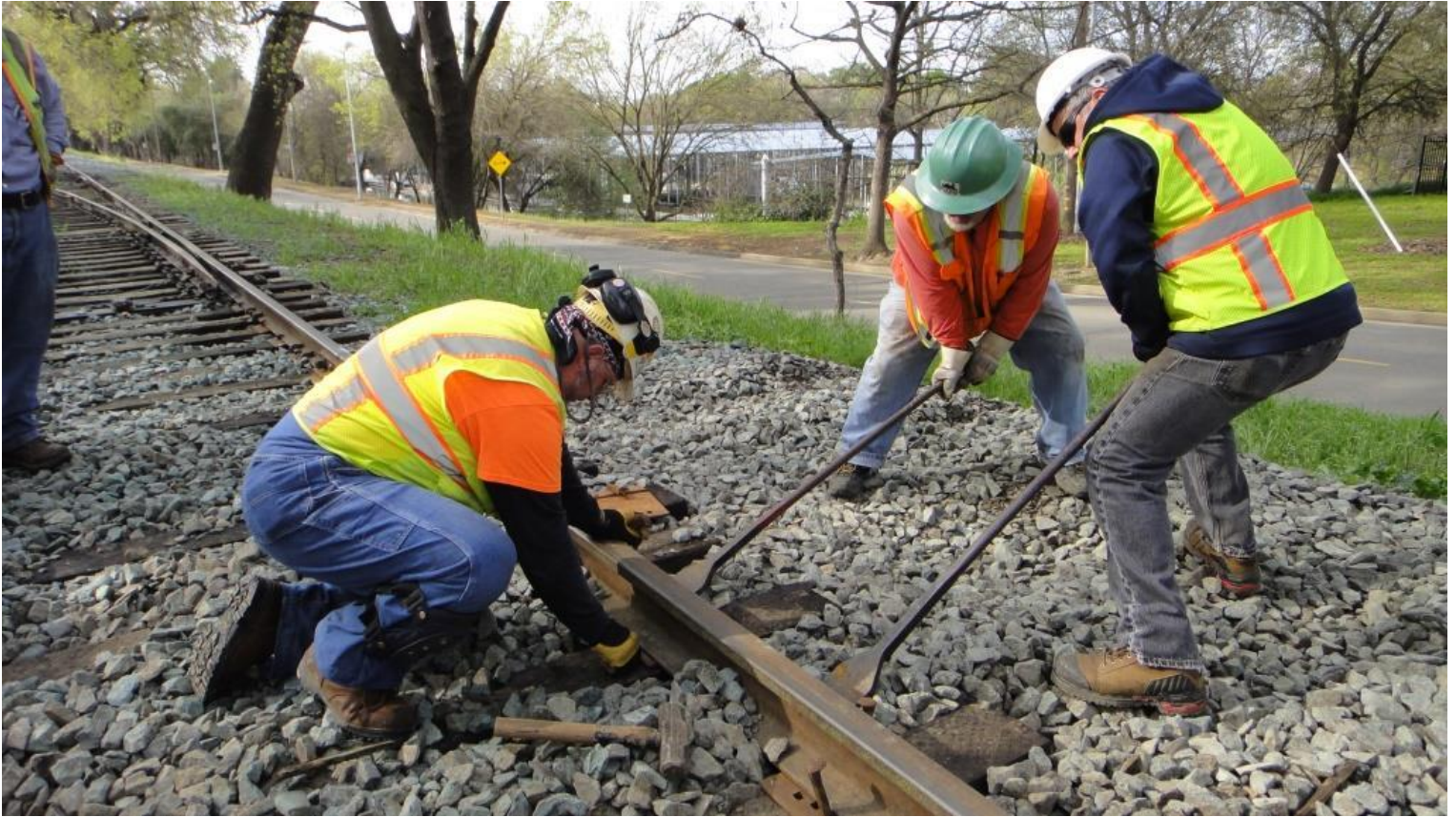
Now Al and Steve nip-up the rail so that Mike F. can squeeze a tie-plate beneath it
