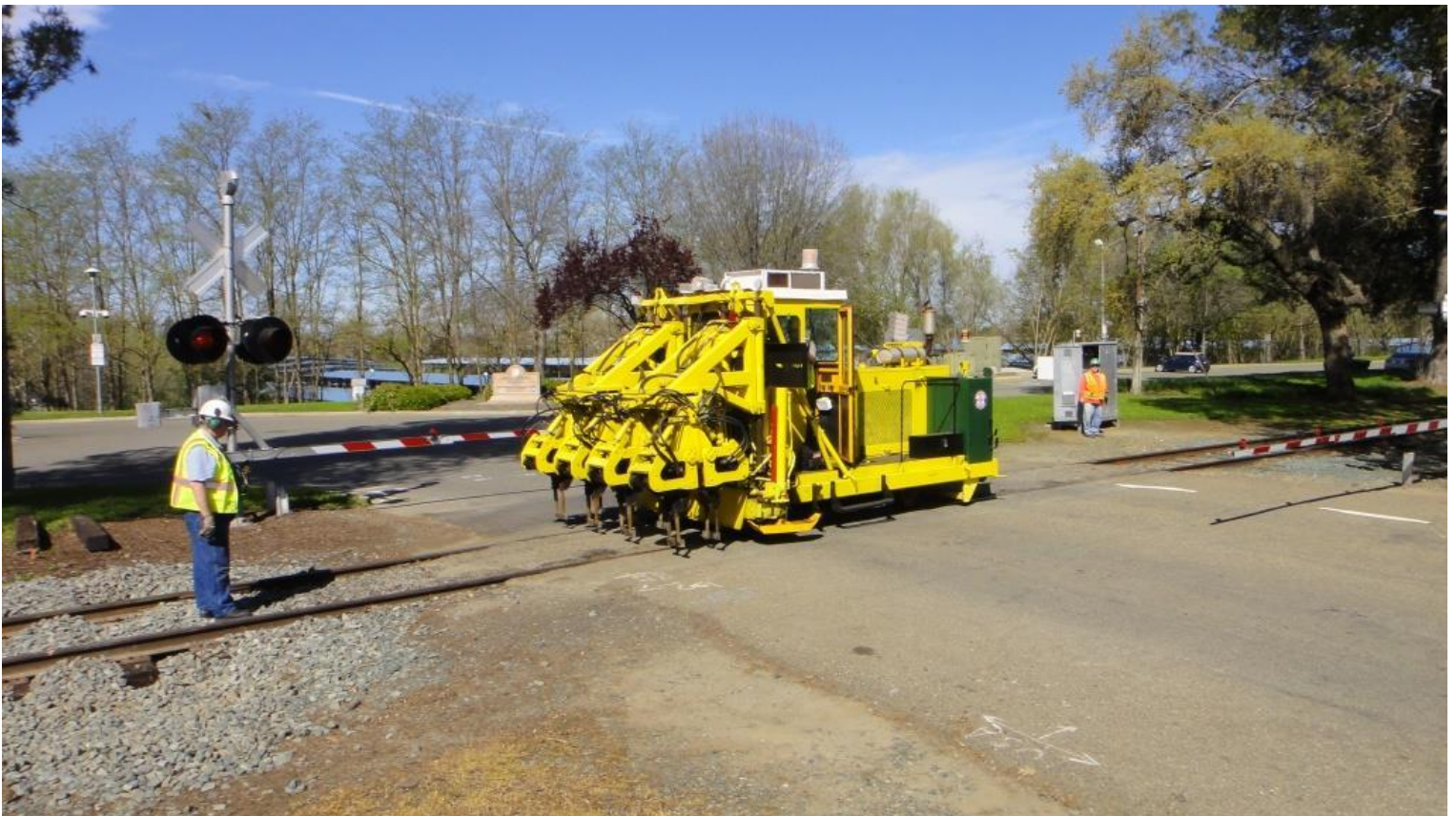
With spiking complete, Heather brings in the tamper. Al activates the crossing gates as Chris C. prepares to guide the tamping action
