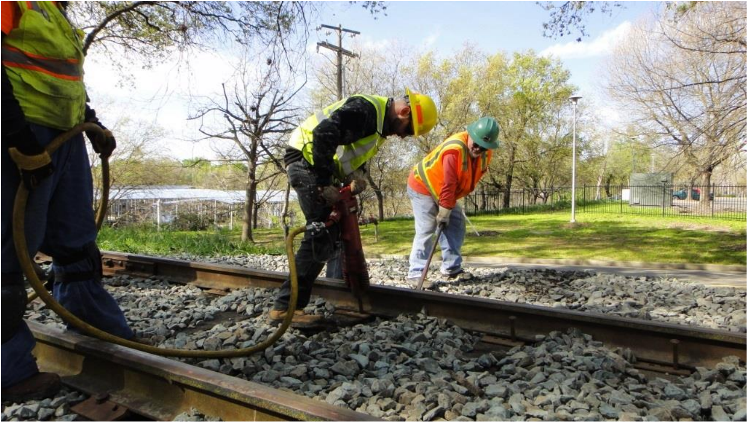
"That's more like it!" With the air-line fully charged, Chris M. drive spikes while Al nips-up the tie
