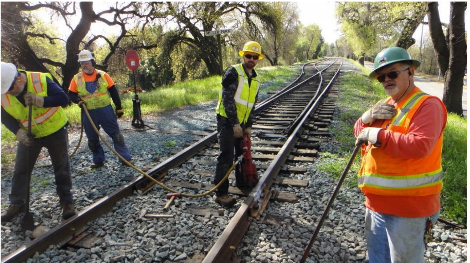
"Where's the air!" Chris M. is all set and ready drive spikes with the pneumatic spike-driver. But, no one turned on the compressor!
